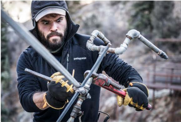
Crew members—including Lucas Carrion, pictured here—fix pipes. XANDER BIANCHI
